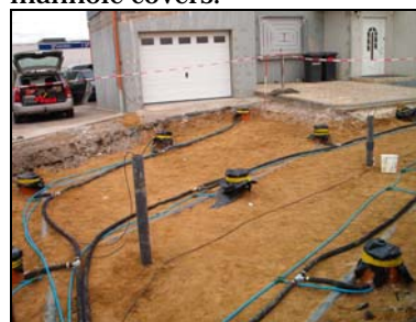
Subsurface electrode/extraction systems
