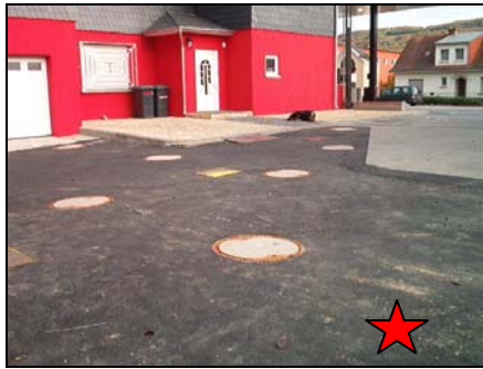
Sub surface finishing of electrodes
